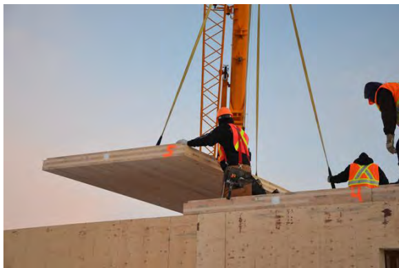
Figure 7: Cross-laminated Timber Panel Assembly, photo by Structurlam 2012.
